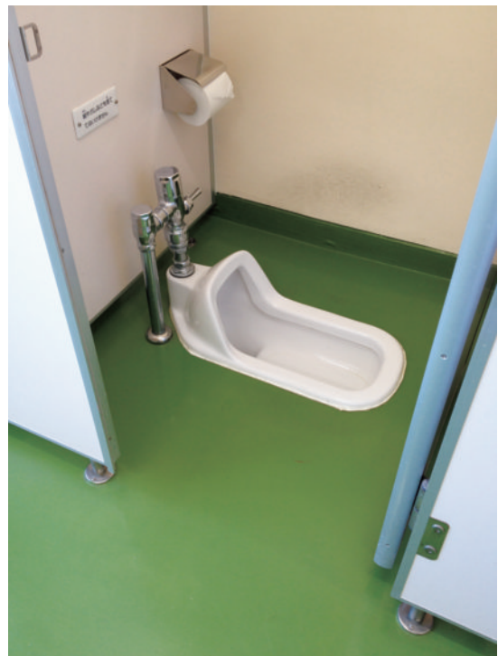
Figure 3 An example of a Japanese-style toilet in an elementary school.
